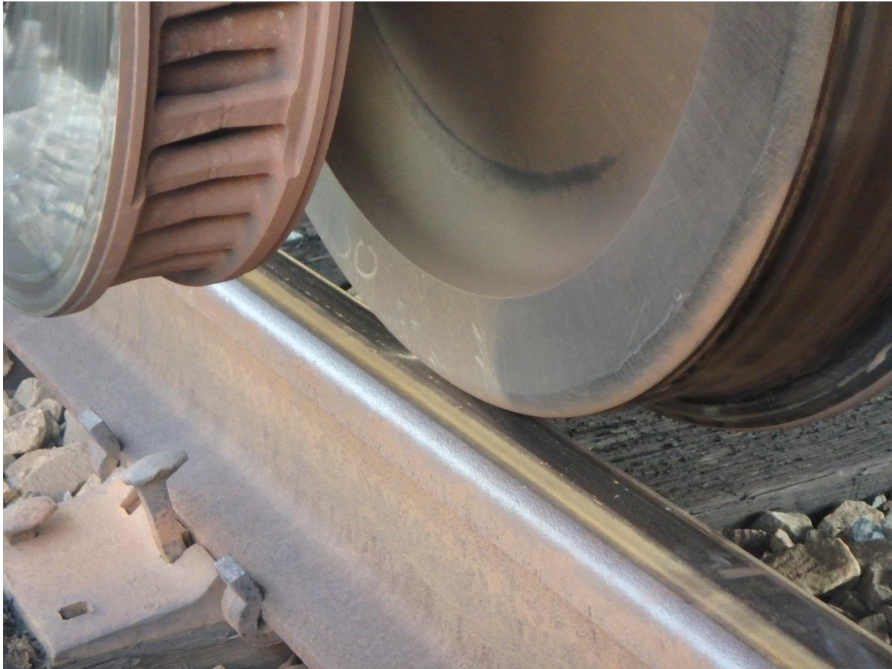
Figure 1. Equipment wheel misalignment and rail head discoloration.
