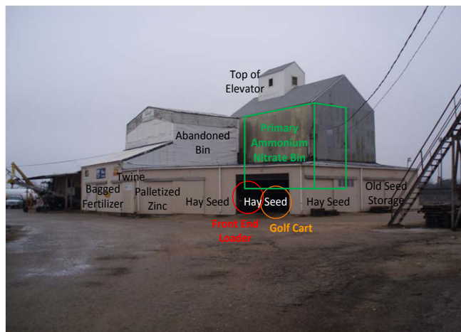
Figure 5. Southwest View from Northeast Corner of Fertilizer Building (Source: WFC Insurer)
