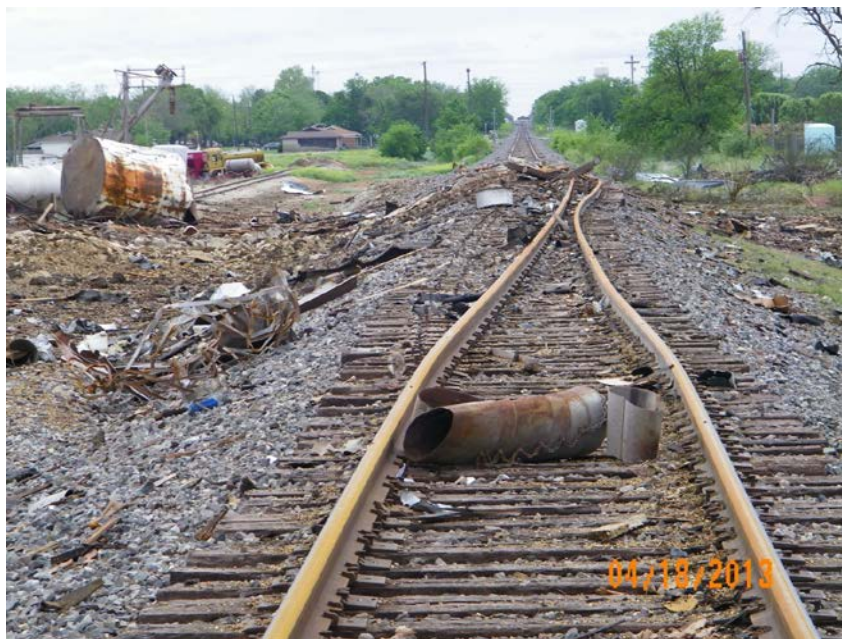
Figure 18. Damaged Railroad Tracks Adjacent to WFC Facility (Source: CSB)
