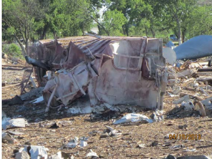
Figure 15. Railcar Loaded with FGAN, Destroyed and Overturned by Explosion (Source: CSB)
