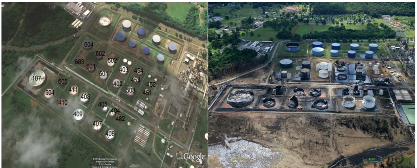
Figure 6: Impact of the explosion and multiple tank fires after the October 23, 2009 incident
