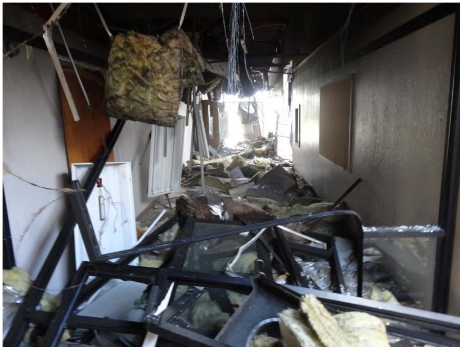
Figure 24. WIS North Hallway, Looking Toward Northeast Exit Door (Source: ABS Consulting)
