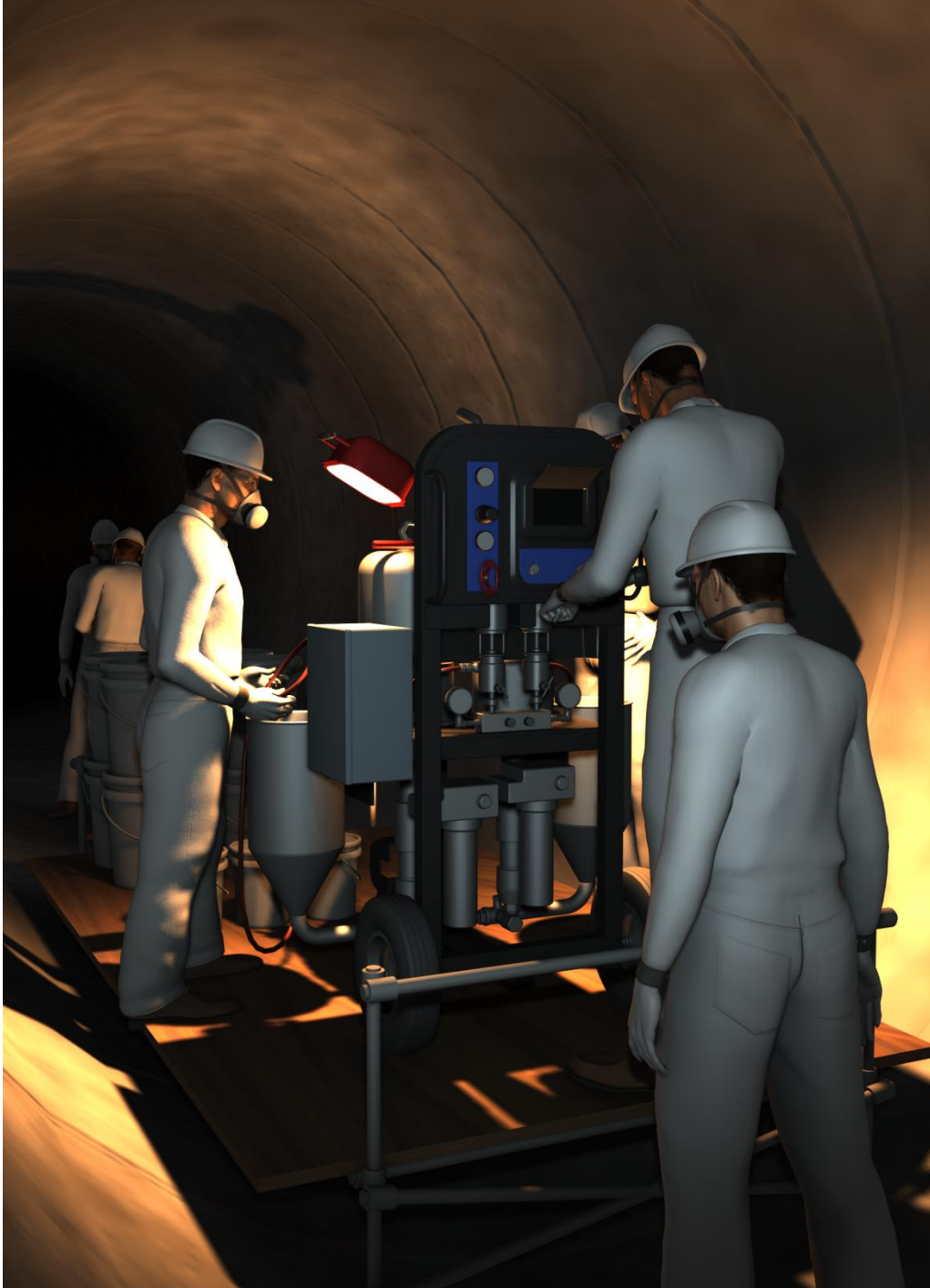
Figure 8. Depiction of contractors working with the sprayer immediately prior to the flash fire
