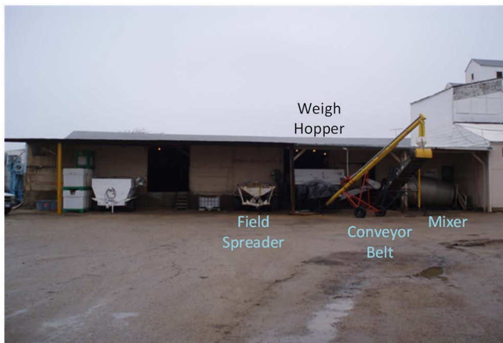
Figure 7. West View from East of Fertilizer Building (Source: WFC Insurer)
