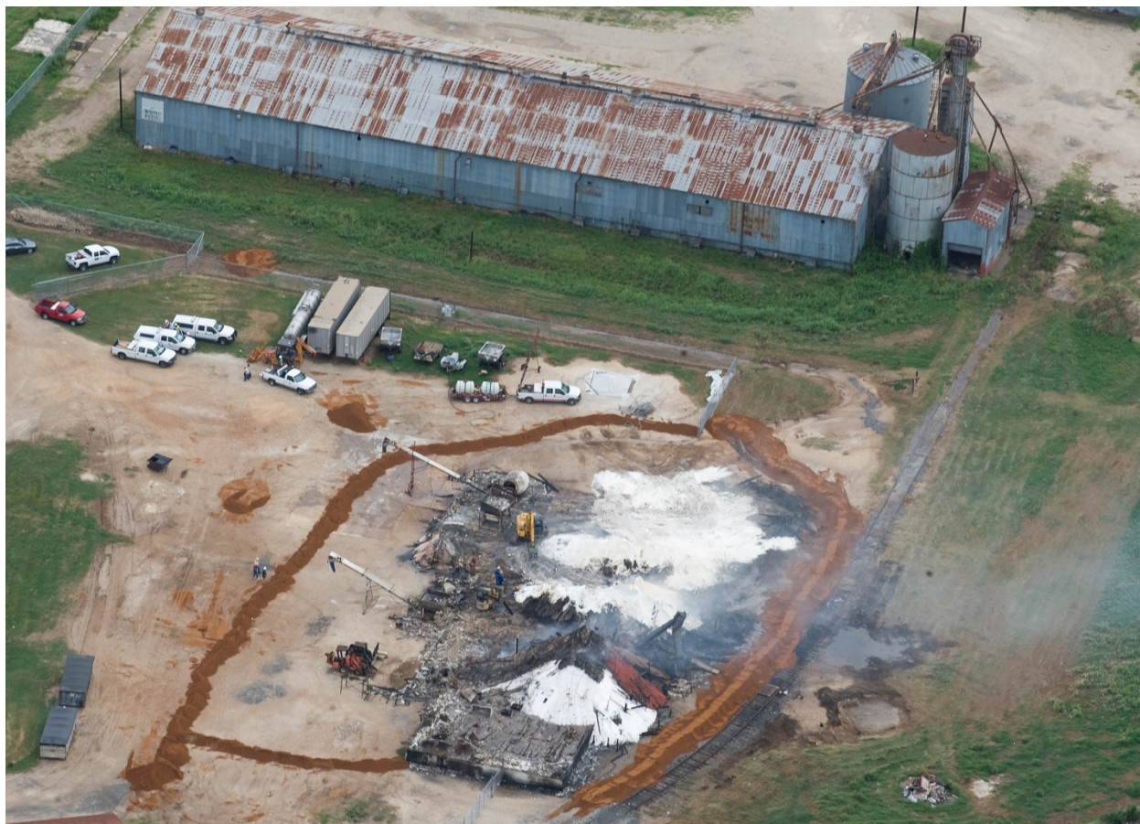
Figure 65. Post-Incident Aerial View of EDC Facility Wooden Fertilizer Warehouse (Source: Bryan-College Station Eagle)
