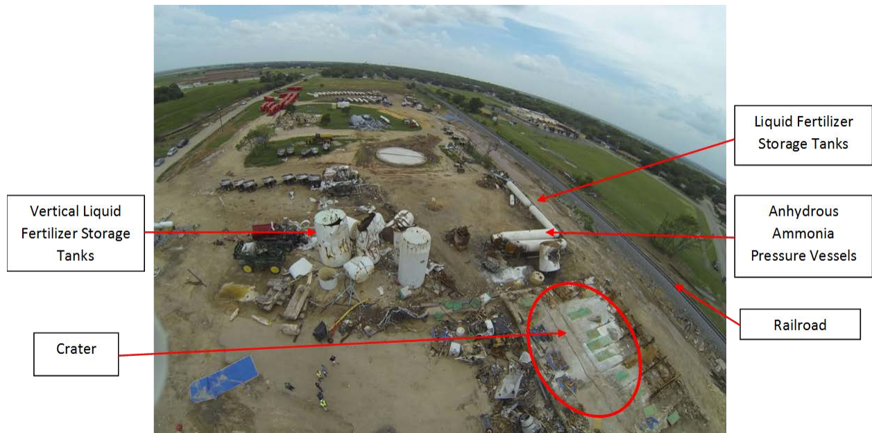
Figure 17. Anhydrous Ammonia Pressure Vessels (Source: CSB)
