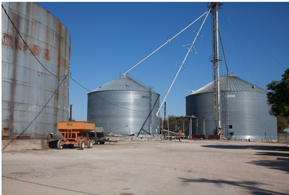
Figure 2. Grain Silos (Source: WFC Insurer)
