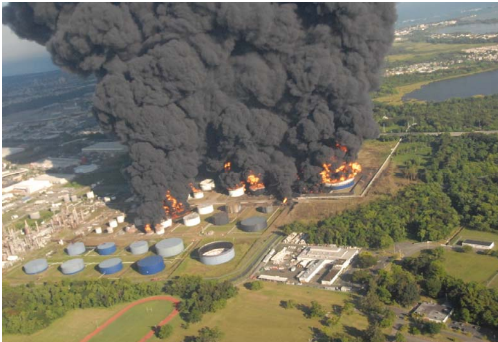
Figure 5: CAPECO multiple tank farm fire, October 23, 2009.
