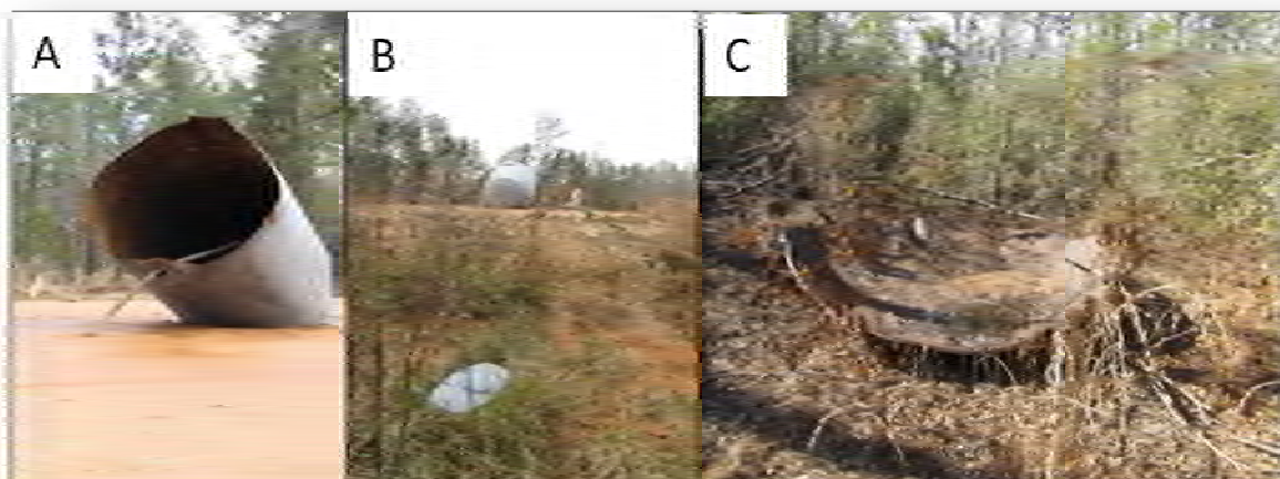
Figure 6-2: A) Remnants of exploding tank B) Tank hatch located approximately 300ft from berm C) Bottom of tank found 60 feet from berm in adjacent wooded area
