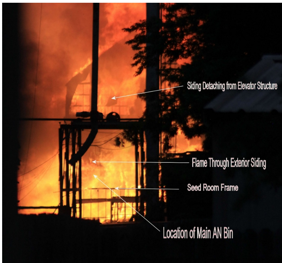
Figure 43. North Side of Structure Approximately 3 Minutes Before Detonation, with Dark Foreground Objects Associated with the Bin Complex North of Fertilizer Building (Source: Member of the Public)
