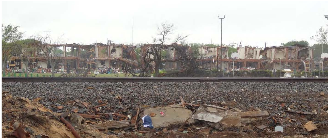
Figure 36. West Terrace Apartment Complex East Façade (Source: CSB)
