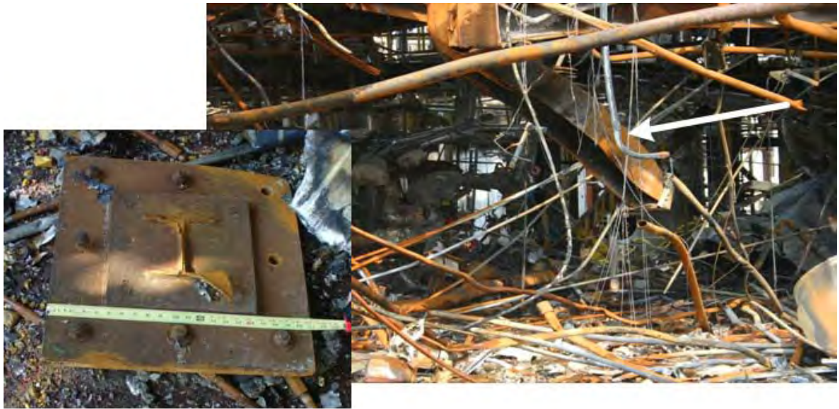
Figure 14. Structural column (arrow) ripped from the steel baseplate (left)
