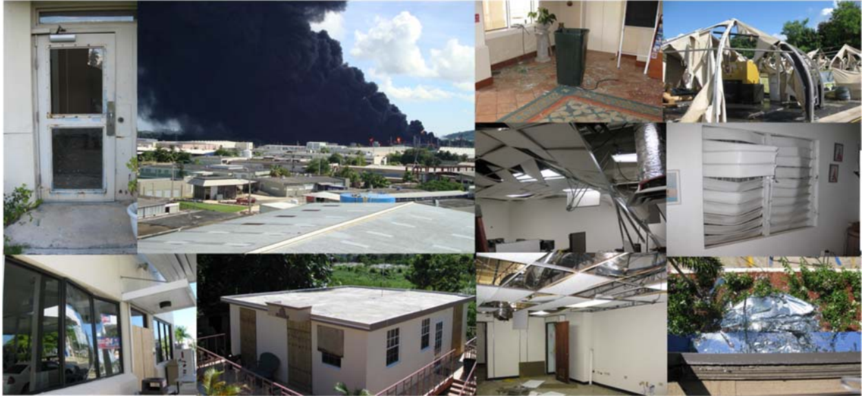
Figure 10: Community damage surrounding the CAPECO facility
