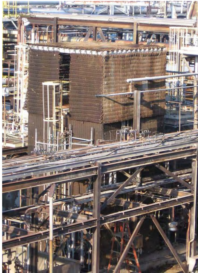
Figure C-2. MIC day tank shield structure
