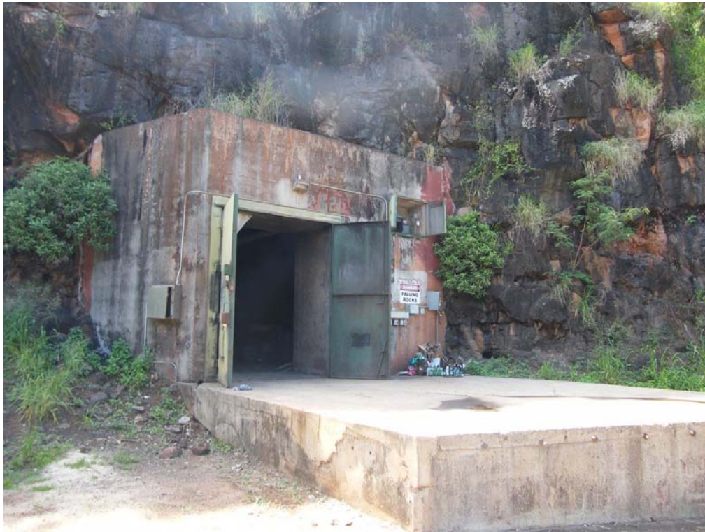
Figure 4. Magazine A-21 (and loading dock), Waipahu, Hawaii
