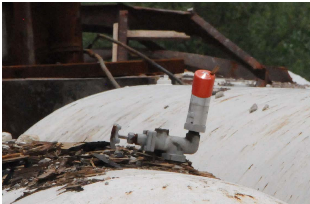
Figure 21. Anhydrous Ammonia Tank PRV, Post-Incident (Source: CSB)
