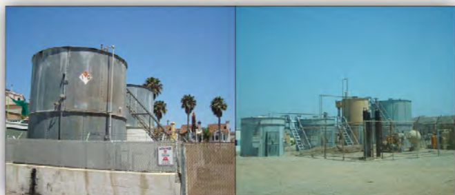
Figure 8-2: Tank battery in Los Angeles, California
