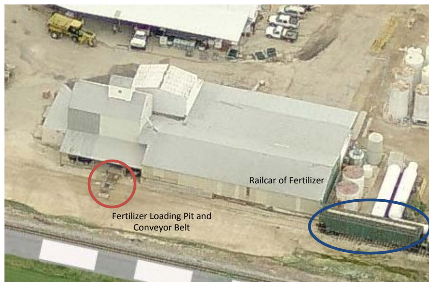
Figure 3. West View of Fertilizer Building (Source: Bing Maps)
