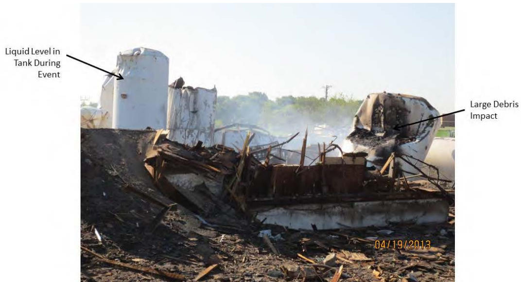
Figure 16. Liquid Fertilizer Tank Damage (Source: CSB)
