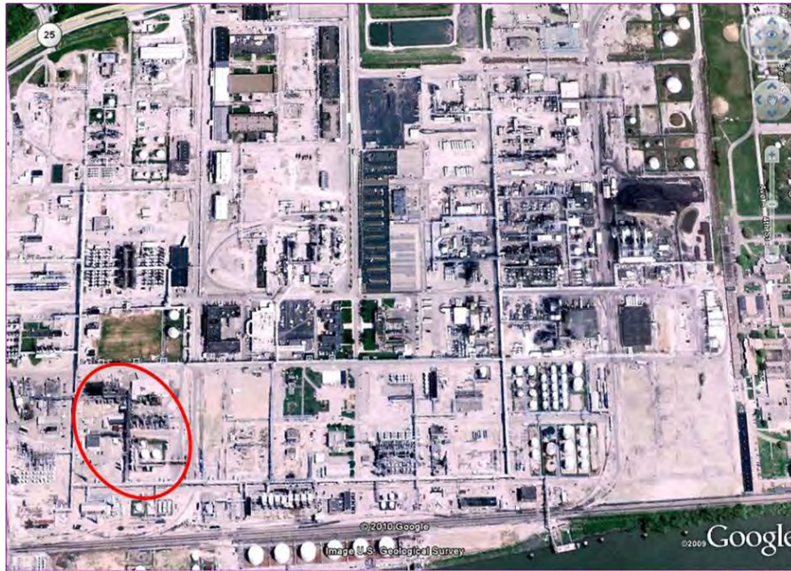
Figure 6. Aerial view of Bayer Institute Manufacturing Park. Methomyl-Larvin unit (circled) is in the West Carbamoylation Complex
