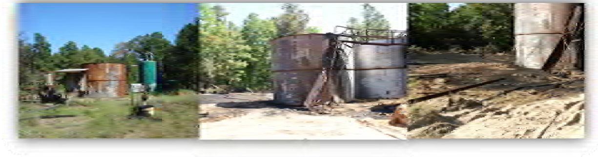
Figure 6-8: MC Production Oil tank site, New London, Texas
