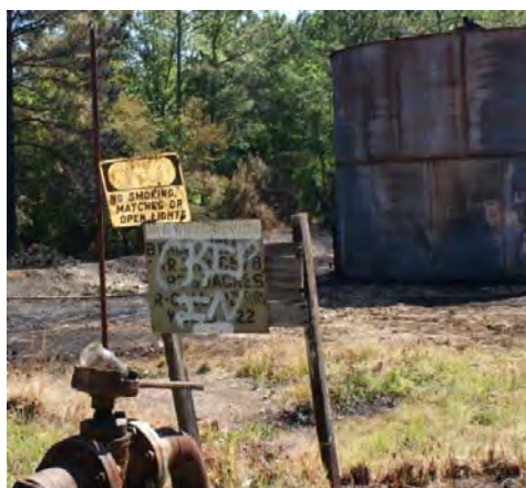
Figure 6-10: M-C Production tank site with warning sign
