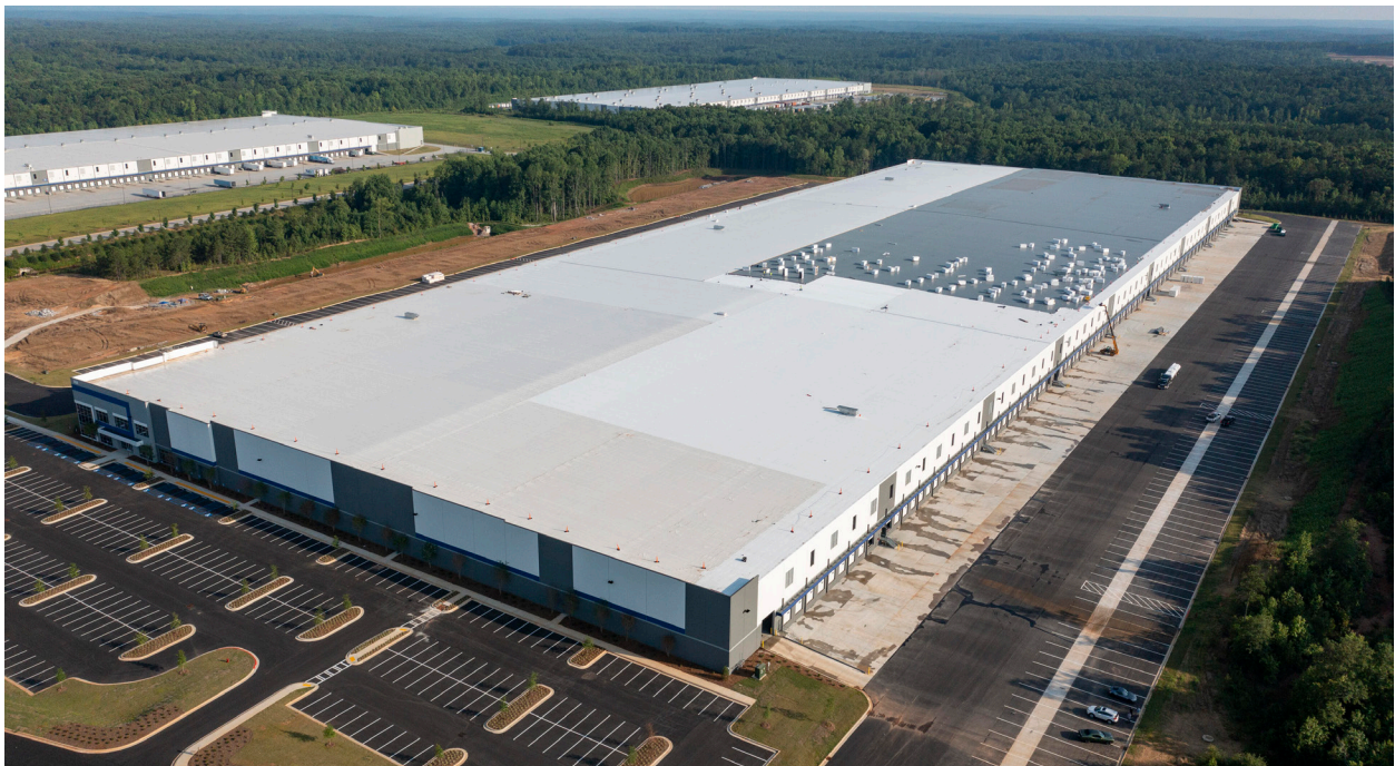
Our new Regional Processing & Distribution Center in Atlanta, GA
